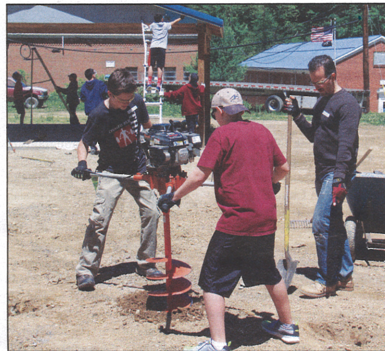
Palatine eighth graders begin construction on a playground in Wheelwright, Kentucky.
